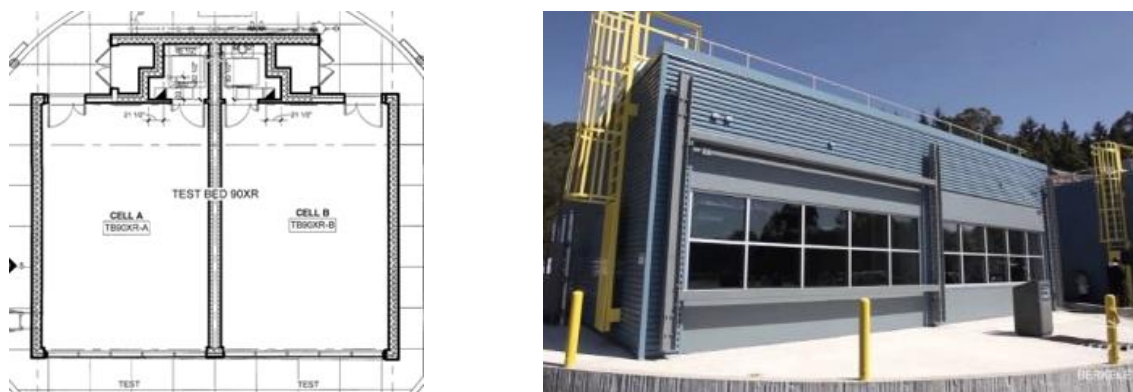
Figure 6 . Floor plan (L) and external view (R) of FLEXLAB testbed showing side by side test cells
